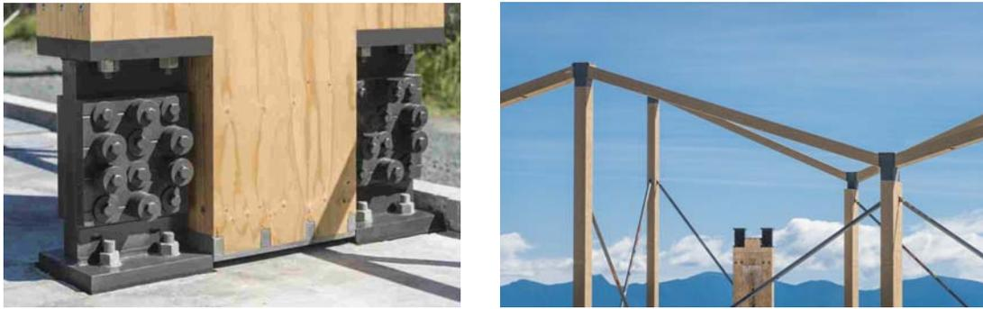
Figure 4. Implementation of the RSFJ technology in the new airport terminal, Nelson, New Zealand
